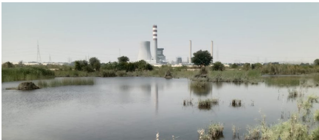
Jamshoro coal-fired power plant, Pakistan. Credit: Zain Moulvi / Alternative Law Collective.
